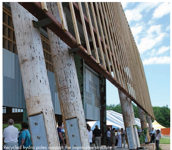
Recycled hydro poles support the impressive structure
